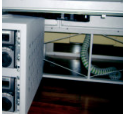
Cable management in a TV studio with triflex® R
